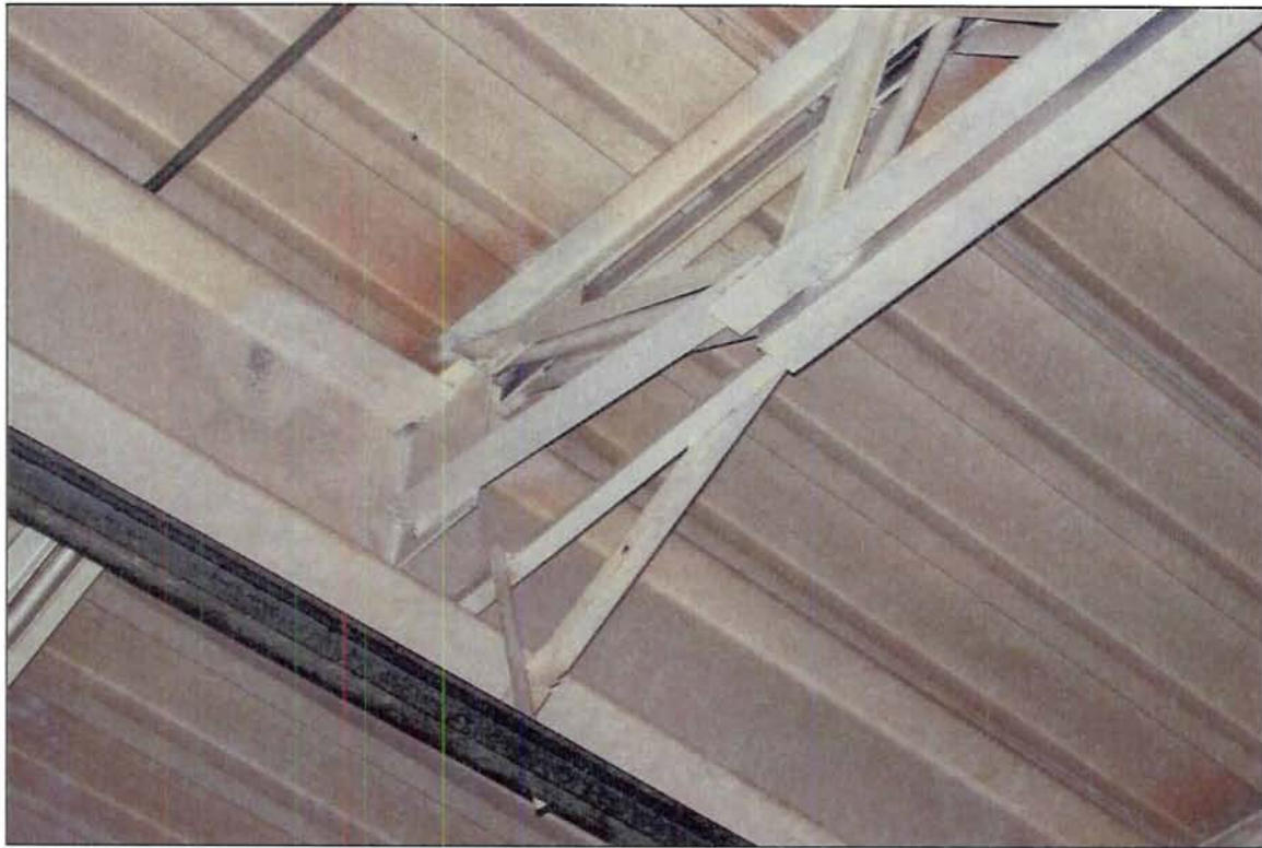
Photo 21 - Typical Joist To Beam Connection
