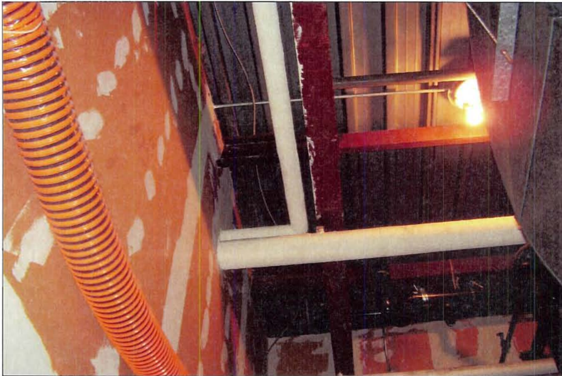
Photo 5 – Exposed Structural Steel Framing In The Mechanical Room
