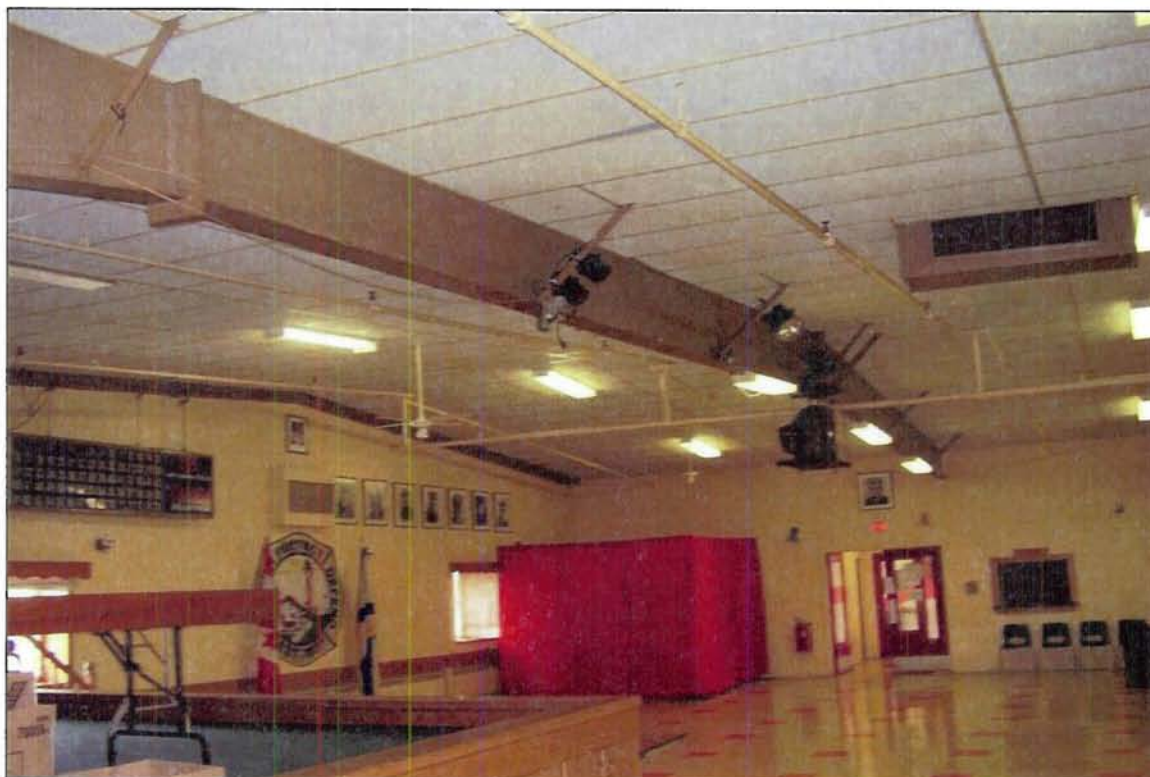
Photo 26 - Second Floor Reception Hall
