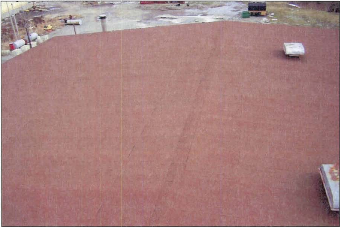
Photo 29 - Typical Condition Of The Roofing Assembly
