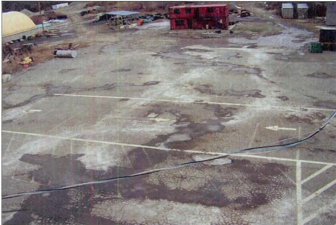
Photo 20 - Overall Condition Of Asphalt Pavement As Seen From The Roof
