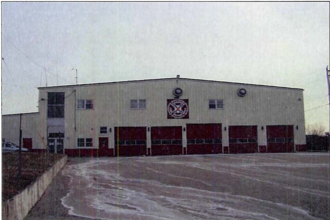
Photo 30 - West Elevation Of The Yarmouth Firehall
