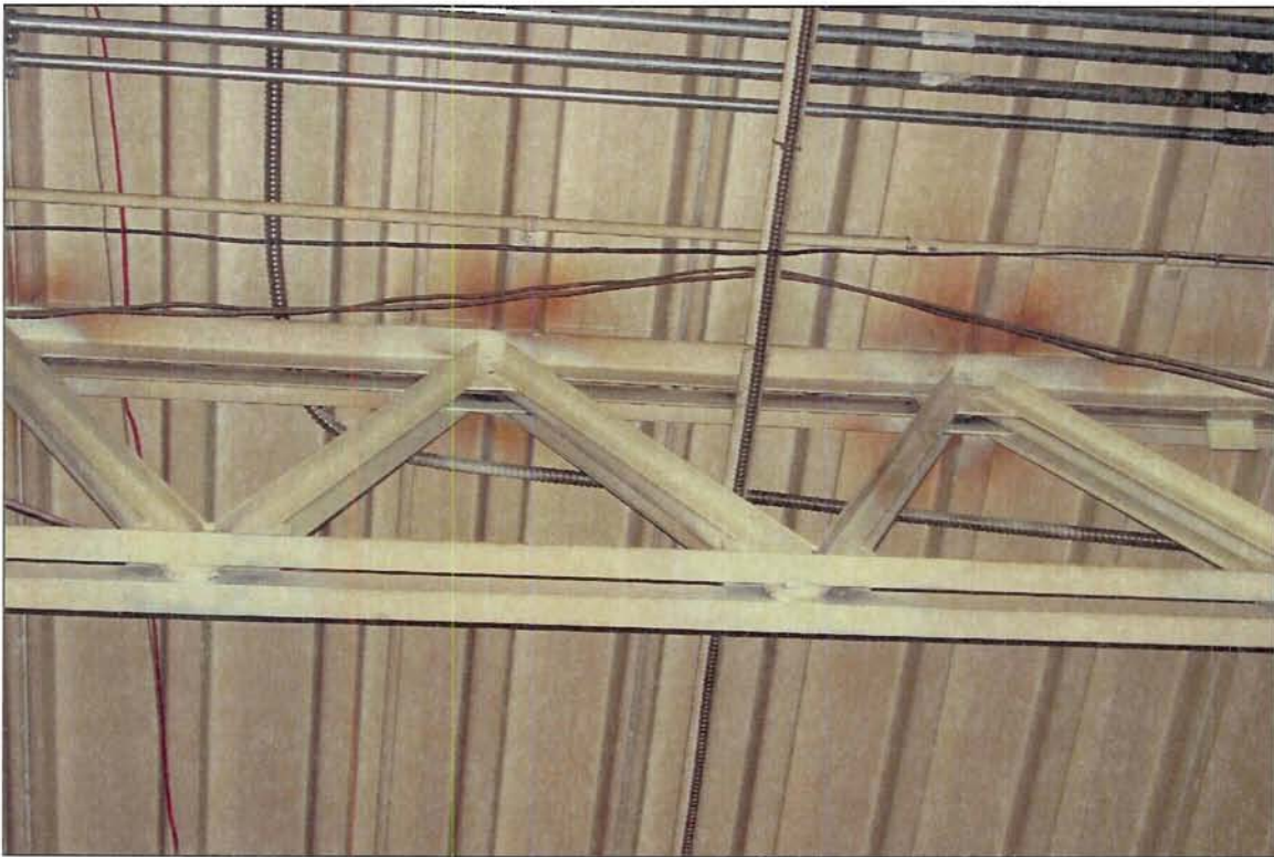
Photo 6 – Typical Open Web Steel Joist In the Truck Bay
