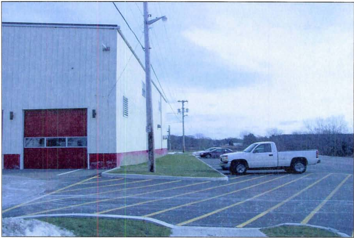
Photo 3 - View Of Exterior Lighting On South Side Of The Building
