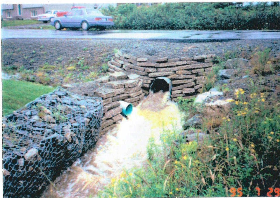
Culvert at Brunswick St - Milo Estates
