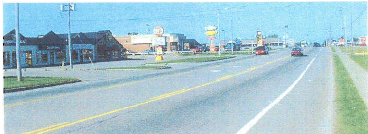
Photo 3.3 - Starrs Road - West of Highway 101 - Urban commercial area.
