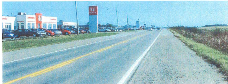
Photo 4.1 - Trunk 3 - the Airport Stretch - east of Hardscratch Road.
