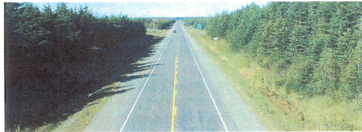
Photo 3.1 - Highway 101 - Westbound approach to Greenville Rd overpass.
