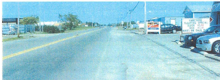
Photo 5.8 - Wide uncontrolled paved entrance, Hardscratch Road.
