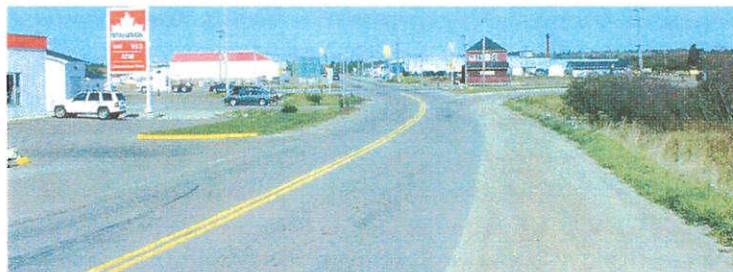
Photo 5.6 - Haley Road - Northbound approach to Starrs Road intersection.
