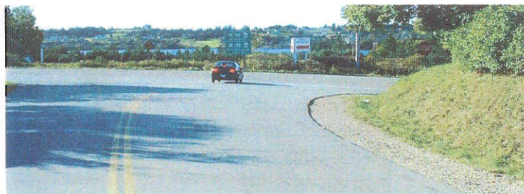
Photo 4.2 - Greenville Road approach to Trunk 1 intersection.
