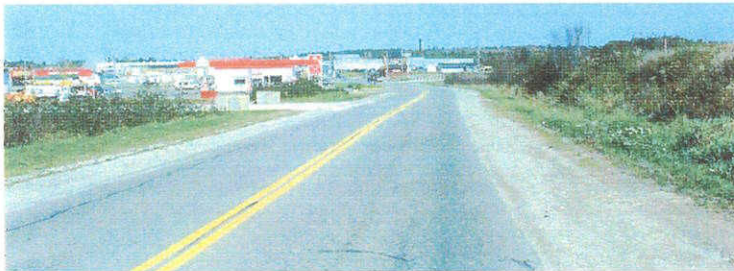
Photo 3.7 - Haley Road - Northbound approach to Starrs Road intersection.
