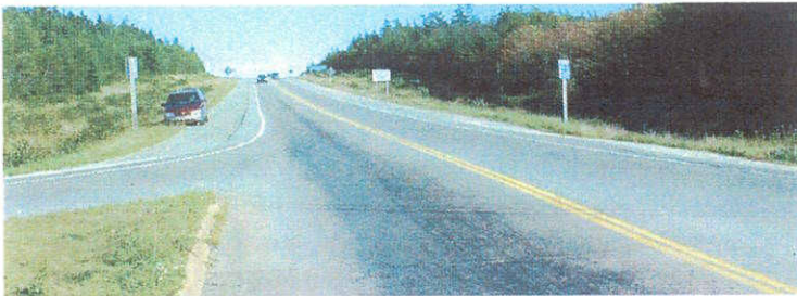
Photo 3.2 - Highway 103 - Eastbound approach to Hardscratch Road.
