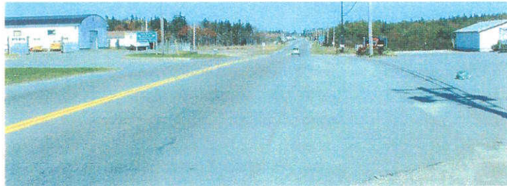
Photo 5.7 - V & R Traps and NSTIR driveways, Hardscratch Road.
