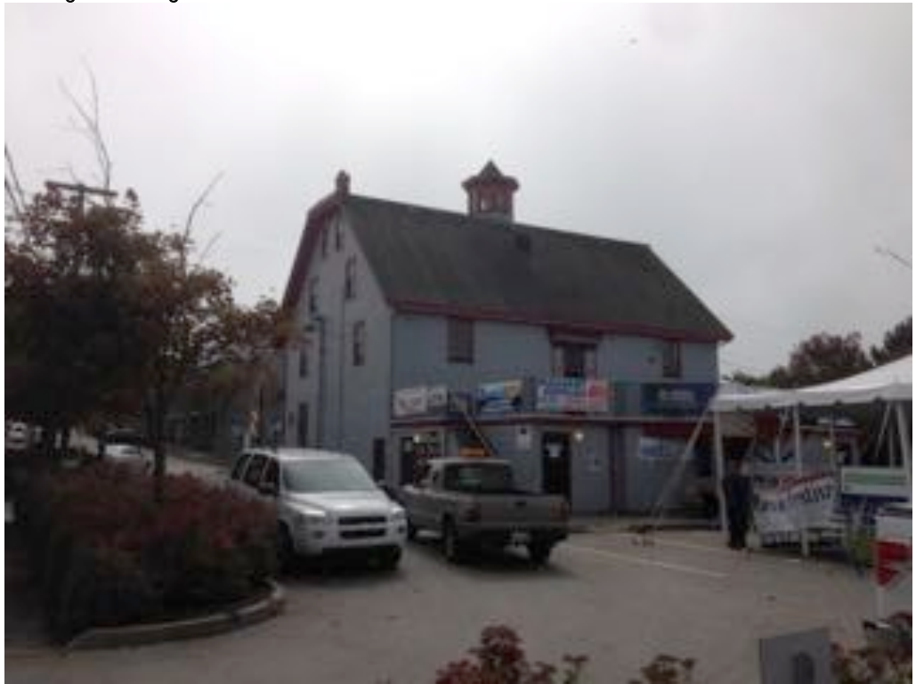
Rear of Killam Wharf Building: note washrooms below and deck above it
