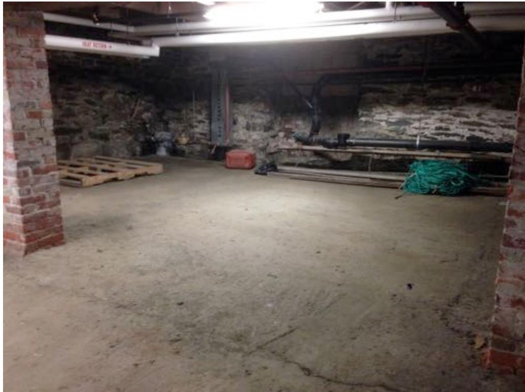
The Basement Has Limited Ceiling Height
