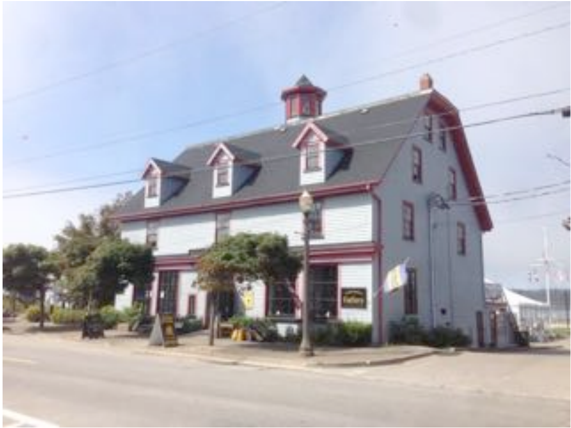
Front of Building from Water Street
