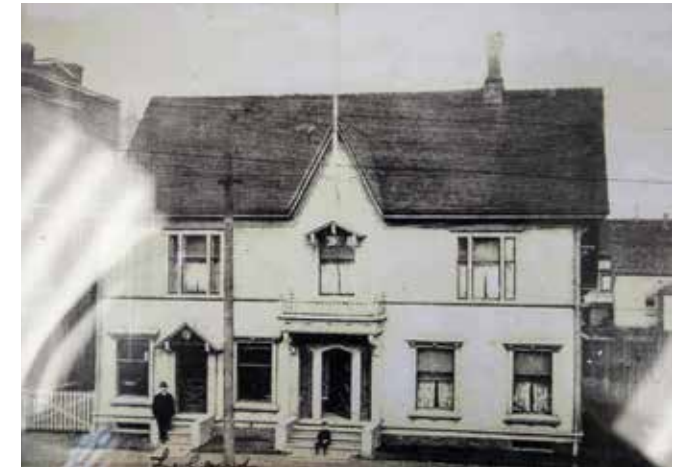
Original building facade
